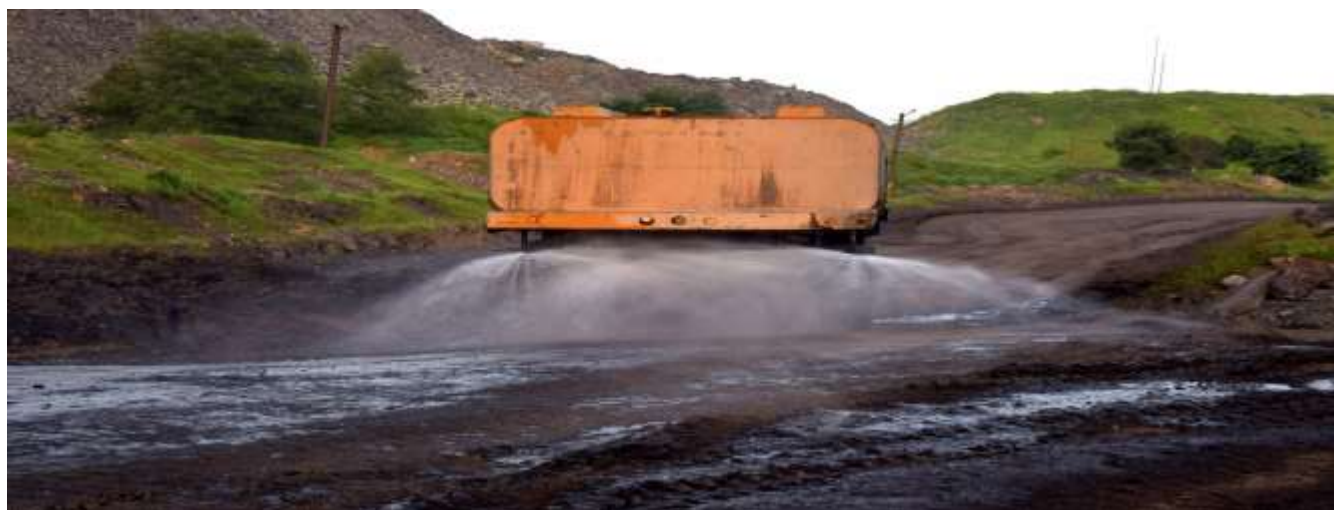
Picture 5.7: A manual sprinkling machine sprinkling water on road
